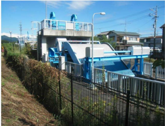
＜七曲川逆流防止樋門＞
