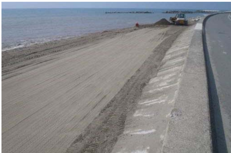
(養浜工施工箇所)
